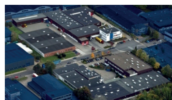
NORD gear factory Glinde
